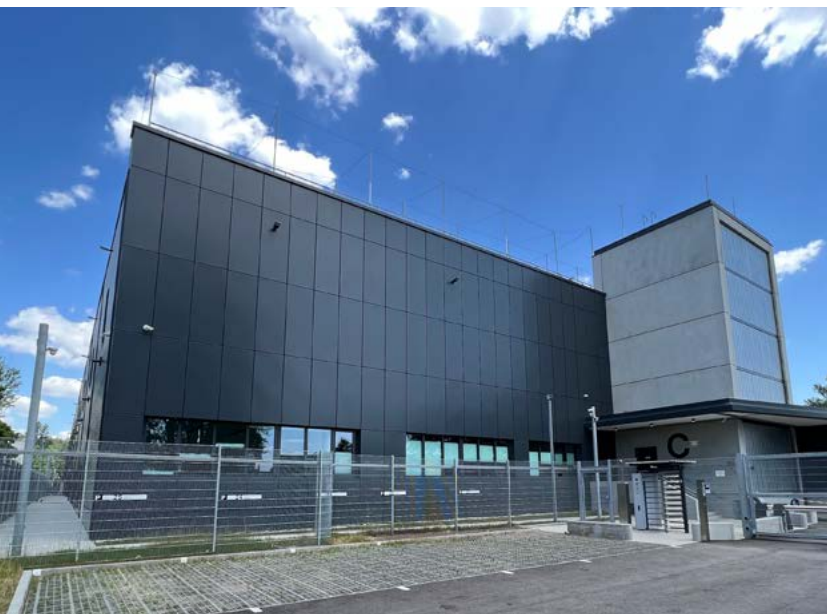
NTT Datacenter, Vienna, AT
