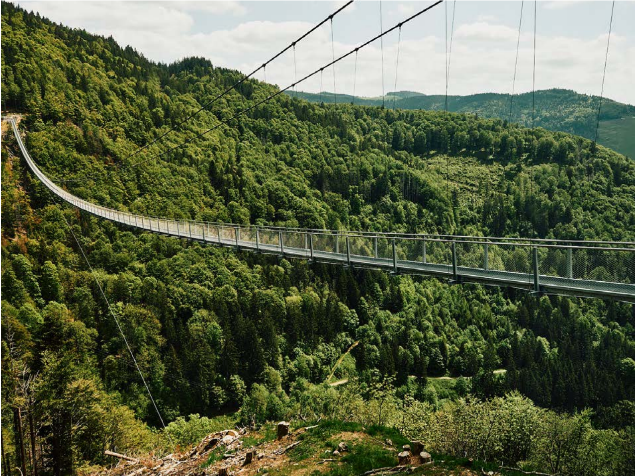
Suspension bridge Todtnau, GER
