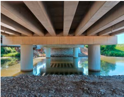
Reconstruction bridge Stretava, SK
