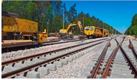
Track doubling, Dobieszyn, PL
