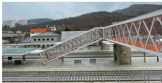
Railroad Crossing Adamov, CZ
