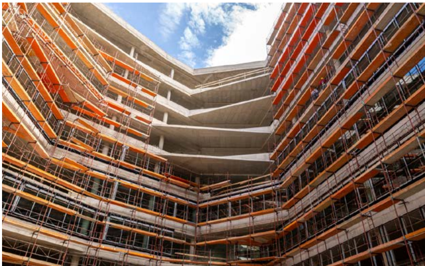
Office Building Liberty, Budapest, HU
