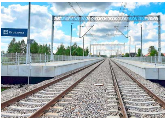
Platforms und track doubling, Kruszyna, PL
