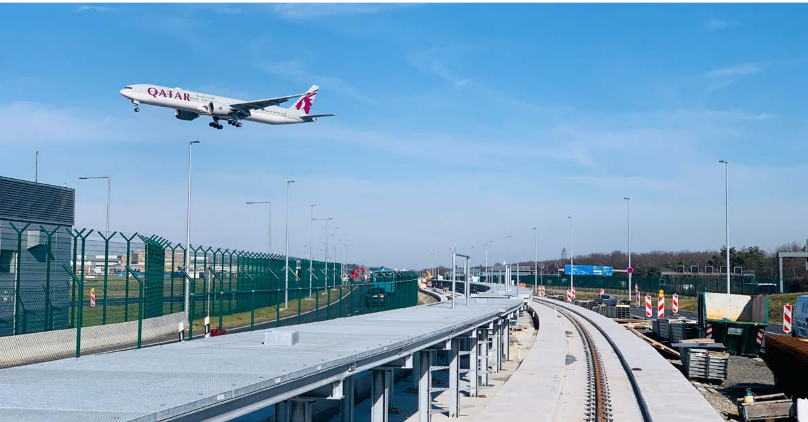
Driving- and power rail assembly, PTS FRA, Frankfurt, GER
