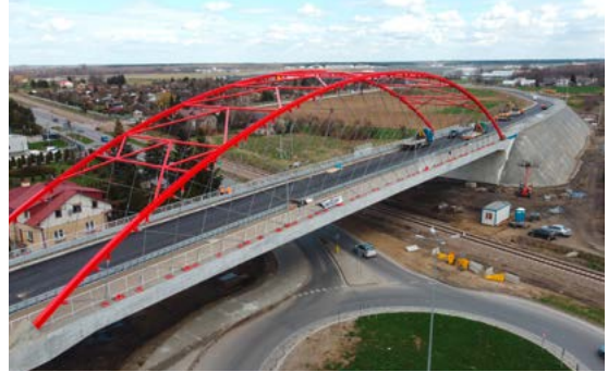
Road and railway viaduct, Mielec, PL
