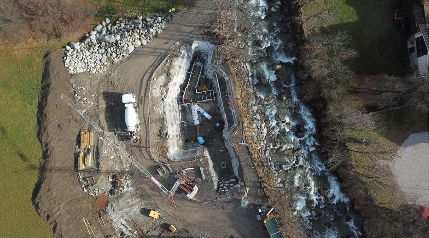
Earthwork unification building power plant Sellrain, AT
