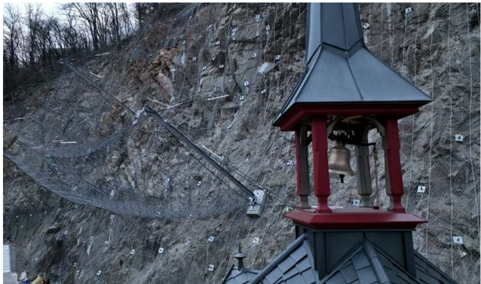
Rock protection Brno, CZ
