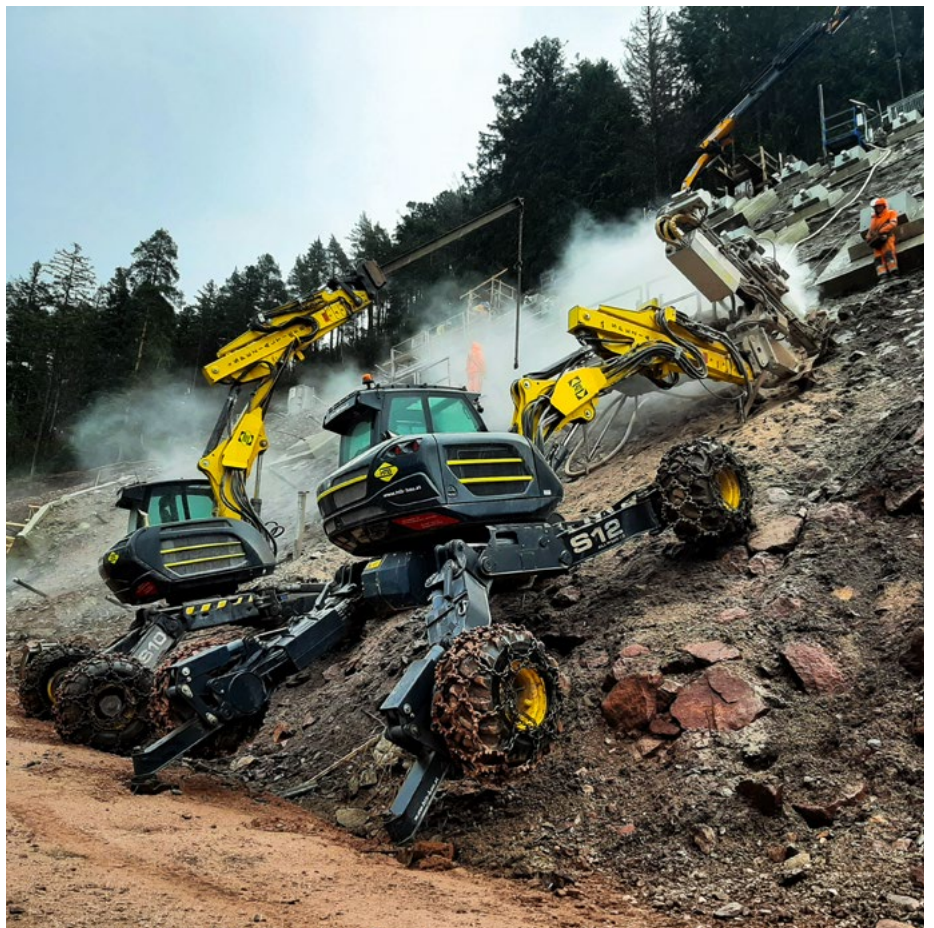
DB Slope Stabilization, Seelenwald, Germany
