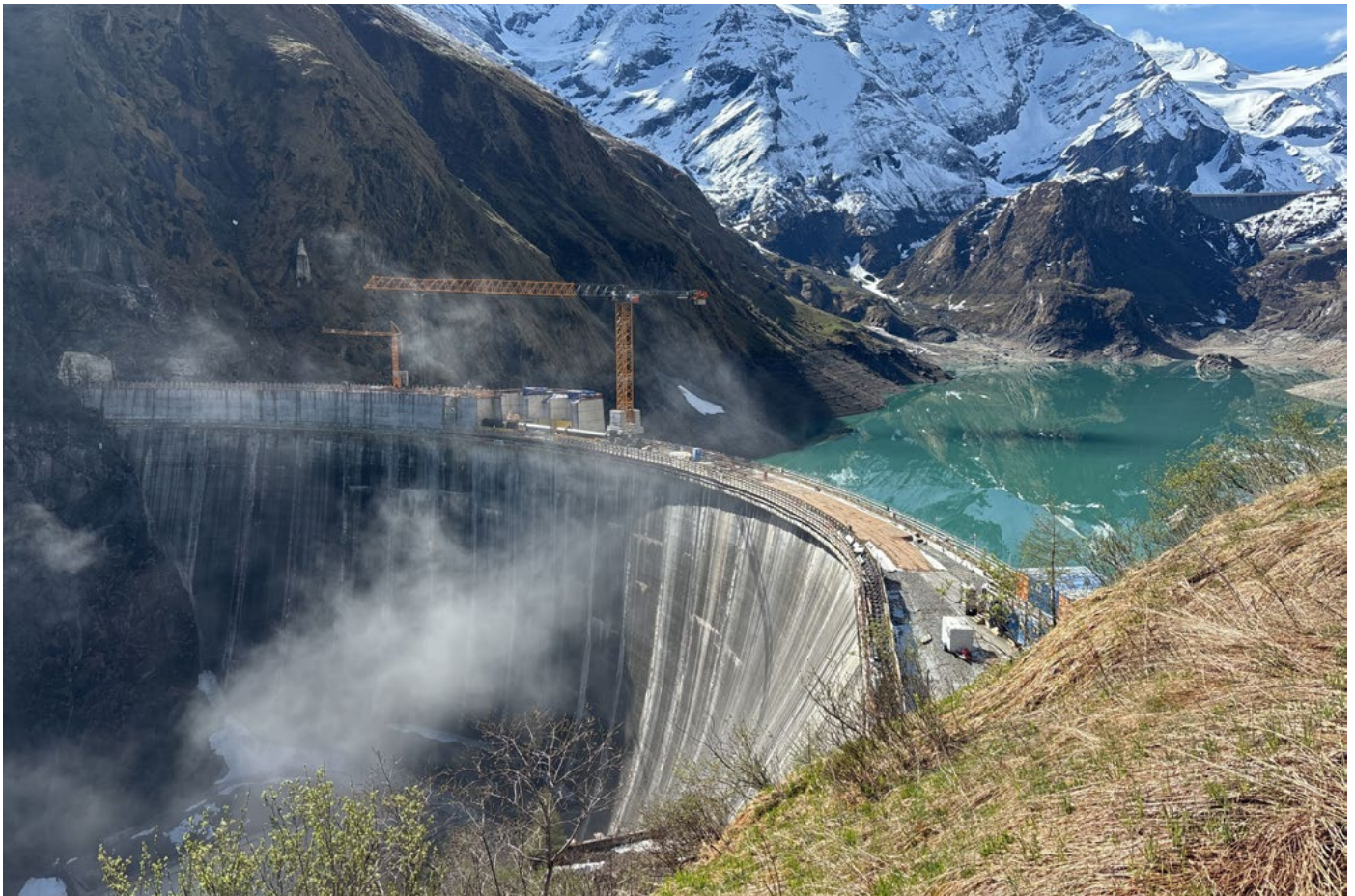
Raising of the Limberg 2 dam, Kaprun, Austria
