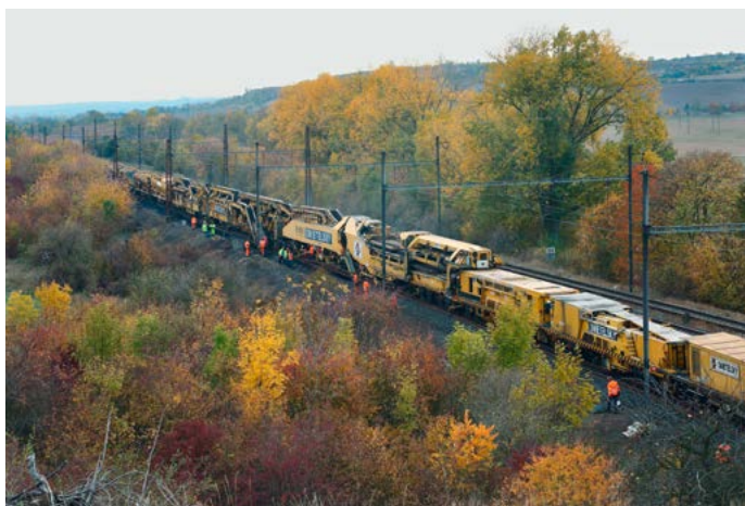
Track construction (RU 800 S), Obrnice – Čížkovice, Czech Republic
